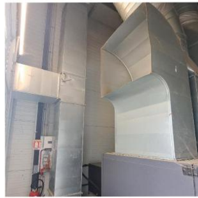
Recovery of heat from the refrigeration unit to be used for heating
