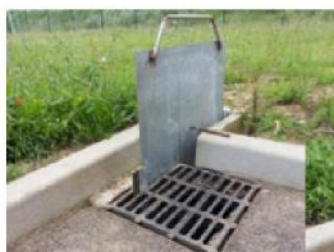
Deep water protection knife gate valve
